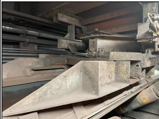
Example conveyor system hopper
