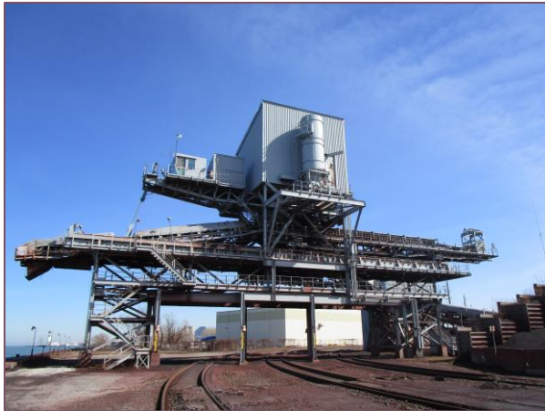
Ship Loader Superstructure
