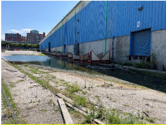
Photo 3.1.3 Large diameter downspouts along NW annex building
