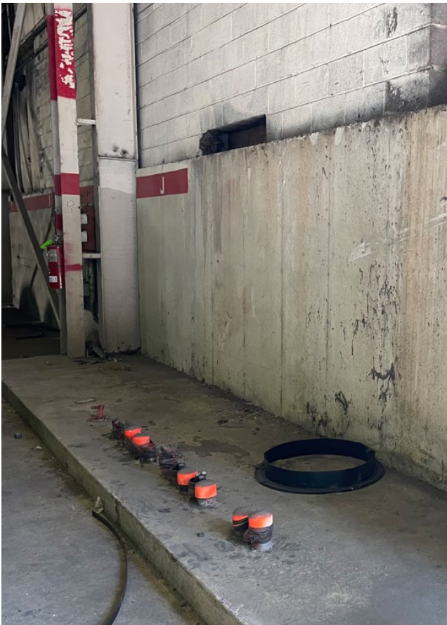
Photo 2.4.2.1 Concrete pad on west side of Warehouse A shows where a main switchboard was demolished
