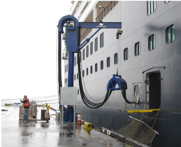
Figure I-5. Fixed and Repositionable Crane Cable Management System
