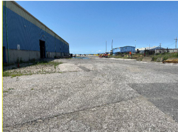
Photo 3.1.4 Condition of pavement along west side
