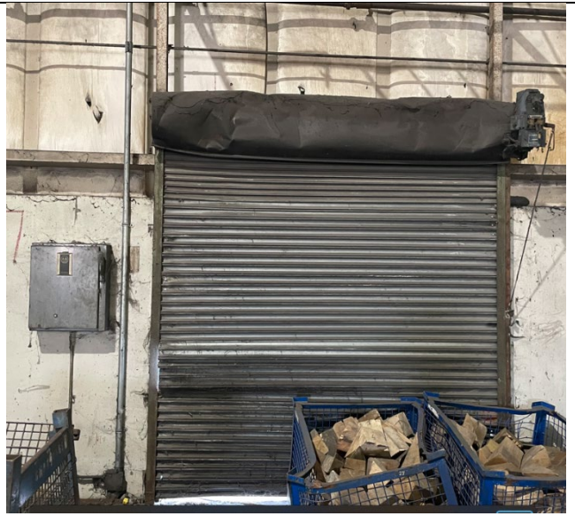
Photo 2.4.2.10 Overhead coiling door on east side of Warehouse, showing A-B starter
