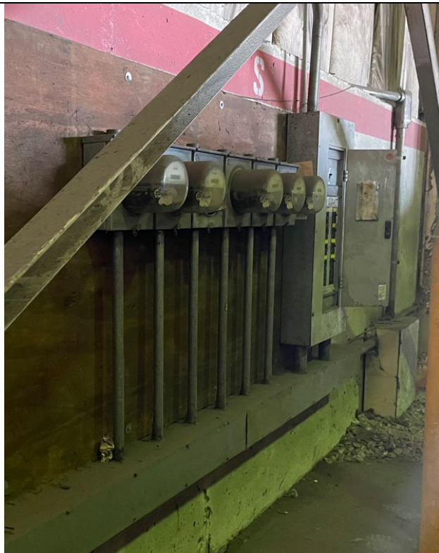
Photo 2.4.2.6 Panel on west side of Warehouse showing energy sub-meters
