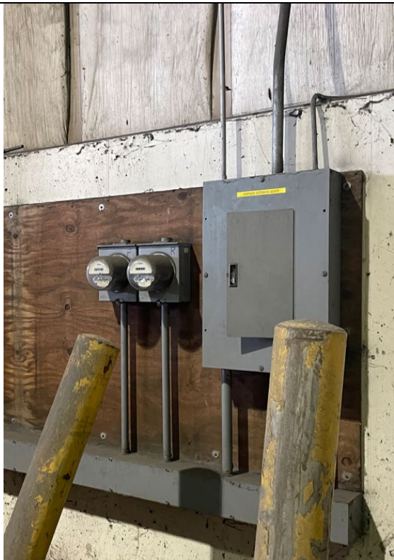
Photo 2.4.2.5 Panel on east side of Warehouse showing energy sub-meters
