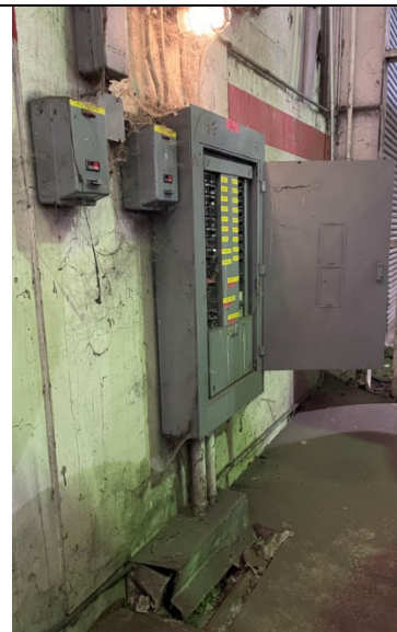
Photo 2.4.2.8 Side view of Panel PA shows where floor at east side of Warehouse A has heaved upwards, crushing wireway below the panelboard
