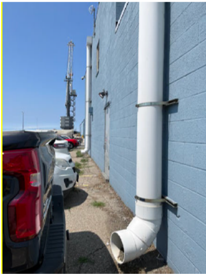
Photo 3.1.3 Large diameter downspouts along NW annex building
