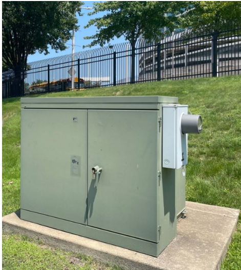
Photo 2.4.1.1 Presence of 12.47kV primary power from CPP occurs on east end of Port Authority site, near W 3 rd St
