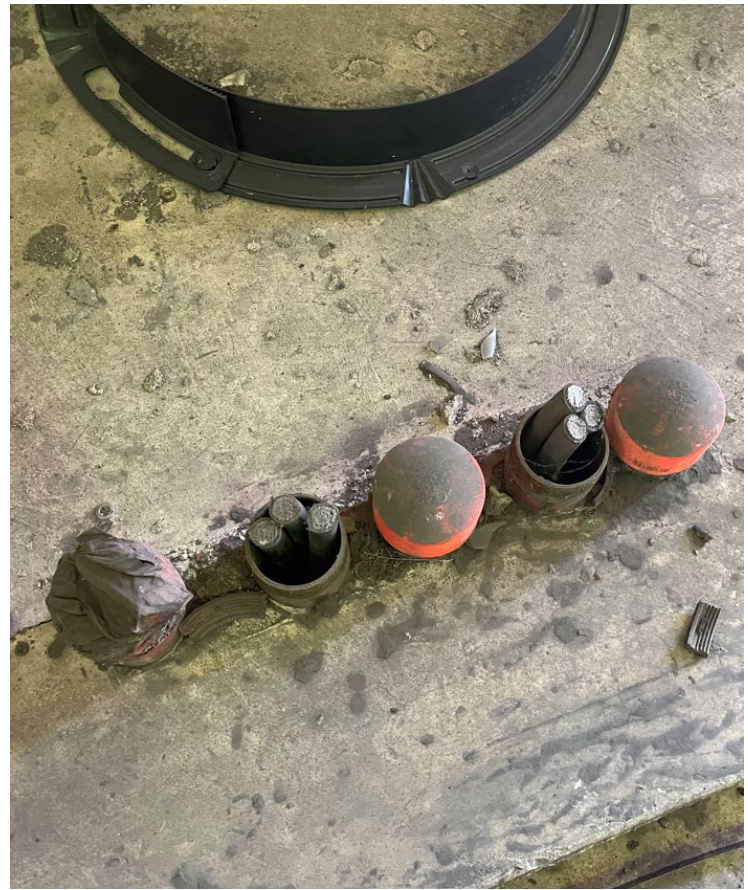
Photo 2.4.2.2 Close-up of conduits through concrete pad for removed switchboard
