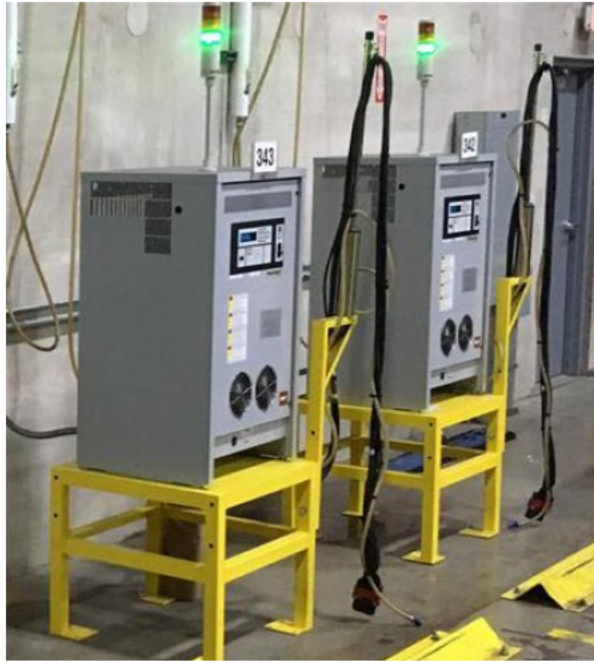
Figure G-3. Posicharge SVS-200 Charging System
