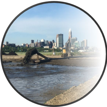
Dredge Material Placement
