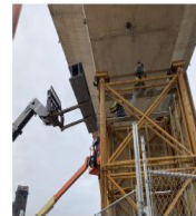
LOCATION OF SEPARATION OF CONCRETE SEGMENTS AND SHEAR CRACKING
