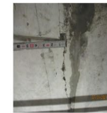
SEPARATION OF BOTTOM FLANGE
