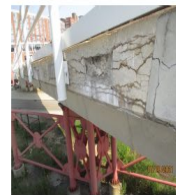
SEPARATION OF BOTTOM FLANGE
