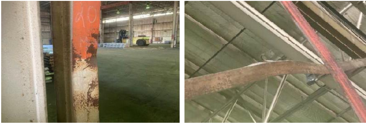
Figure 8: Impacted Column and Cross-Bracing in Warehouse A
