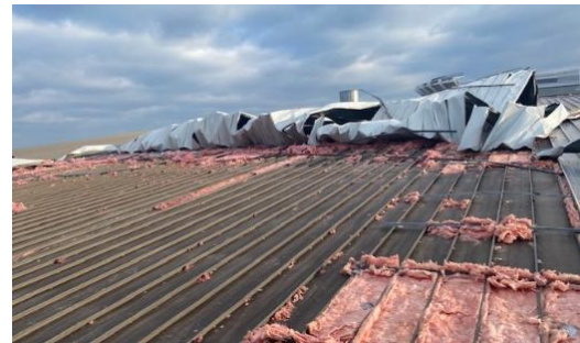
Figure 9: 2021 Warehouse A Roof Damage
