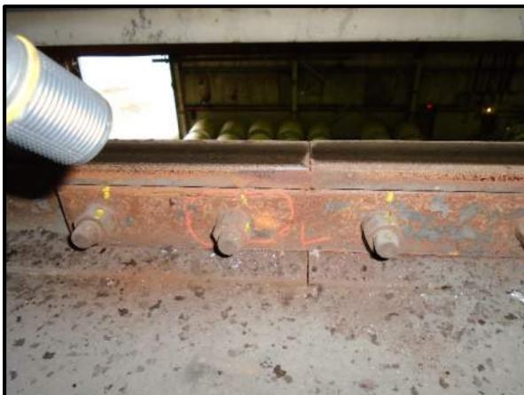
Figure 14 – Match-marked bolts at splice plate
