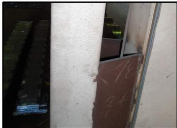
*Figure 6 – Typical plates welded to column flanges*
