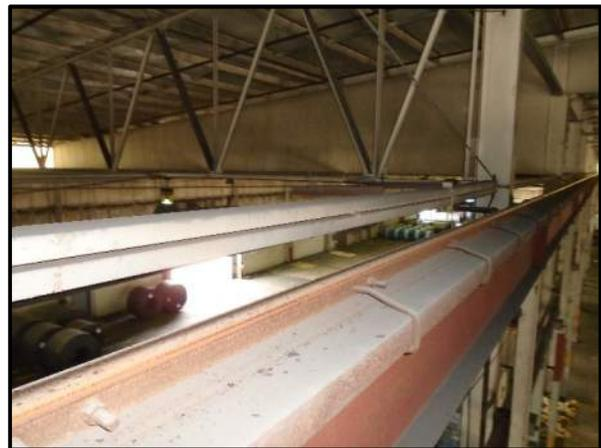
Figure 13 – Typical channel section with crane rail
