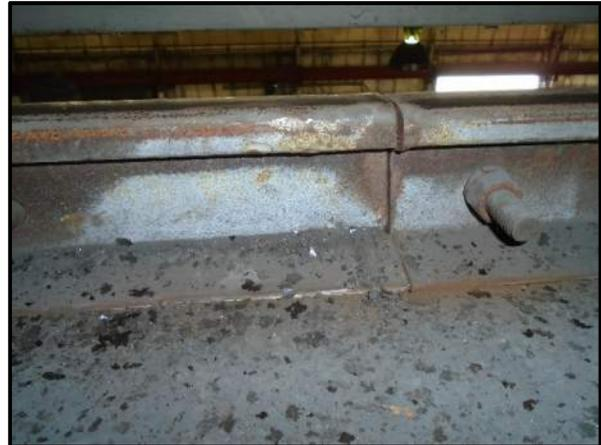
Figure 15 – Missing splice plate at W12-13
