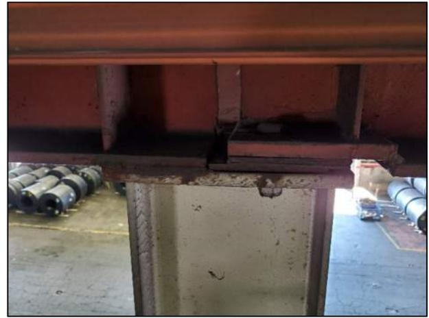
Figure 16 – Loose bolt and missing bolt (left) and bearing connection detail (right)
