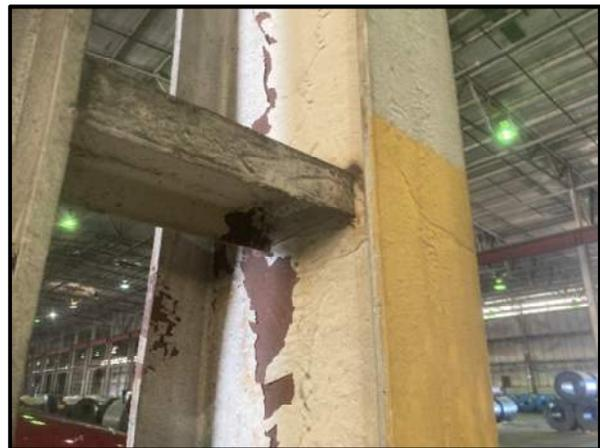
*Figure 4 – Typical channel section welded to column*
