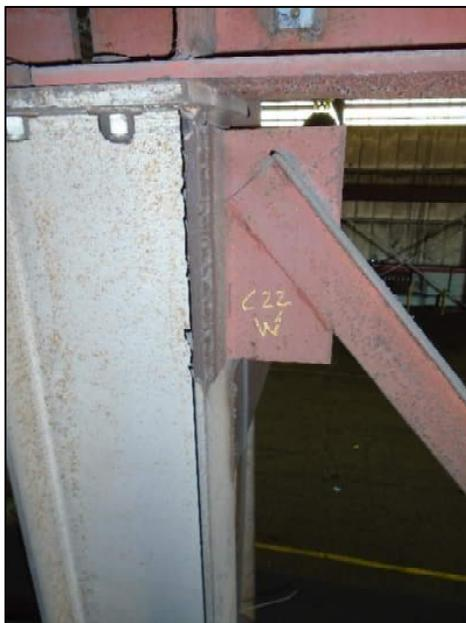
Figure 8 – Typical gusset plate at column
