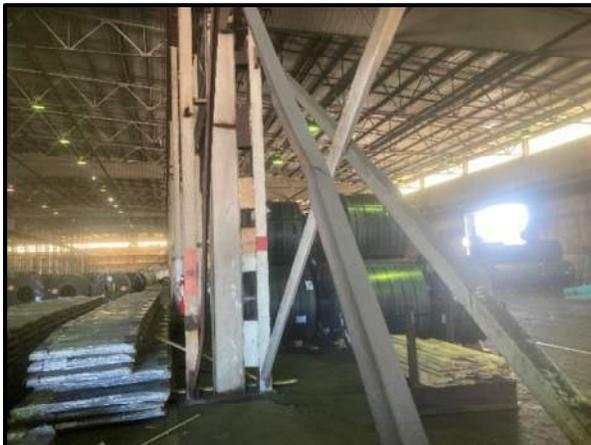
*Figure 5 – Typical cross-bracing*
