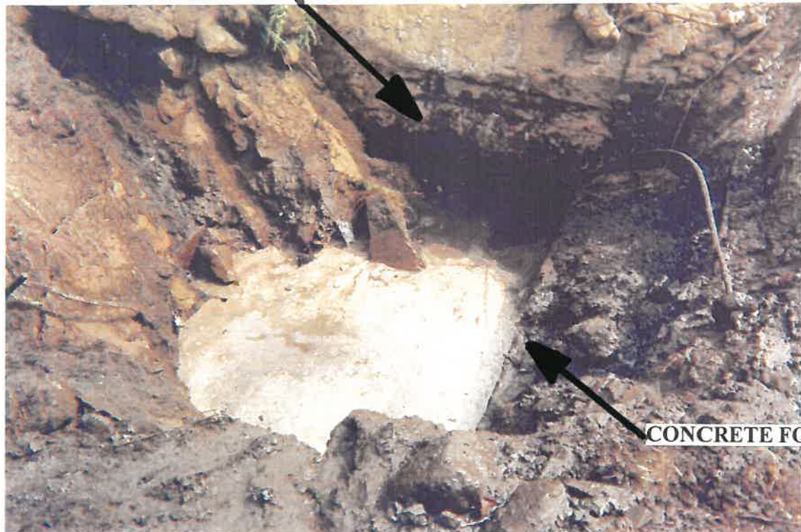
Photo 12: View of northeastern portion of test trench #2 (TT-2) standing approximately 92' east of boring WC-10 looking northwest. The concrete in the upper part of the picture is the western face of the exposed concrete dock. Note concrete footing under dock.
