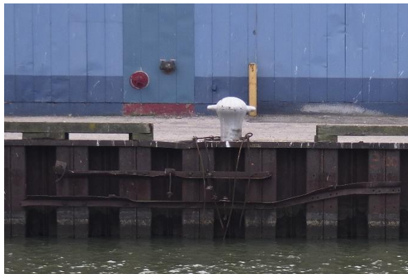
Fig. 13 – Damaged fender system
