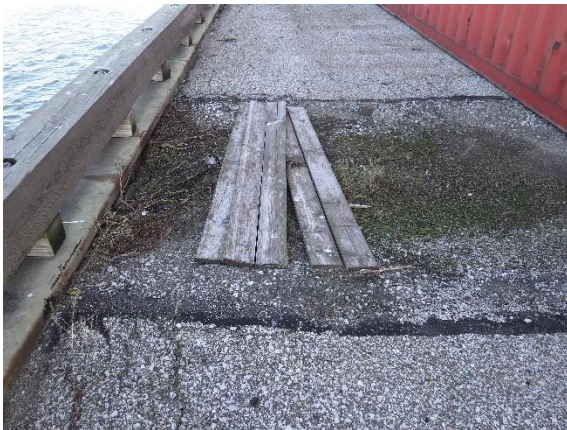
Fig. 1 - Pavement settled and damaged (drainage outlet)
