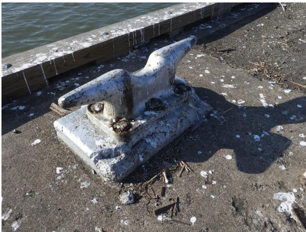
Fig. 9 – Deteriorated mooring cleat foundation
