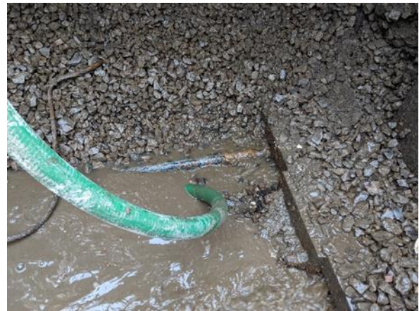
Fig. 18 – Tieback and Waler Exposure
