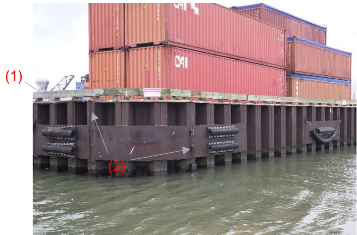
Fig. 4 – Damaged fender (1) and failed connection (2)
