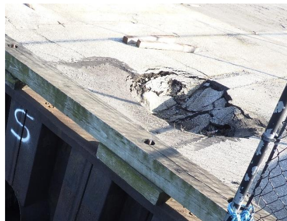
Fig. 16 – Sink hole behind south headwall
