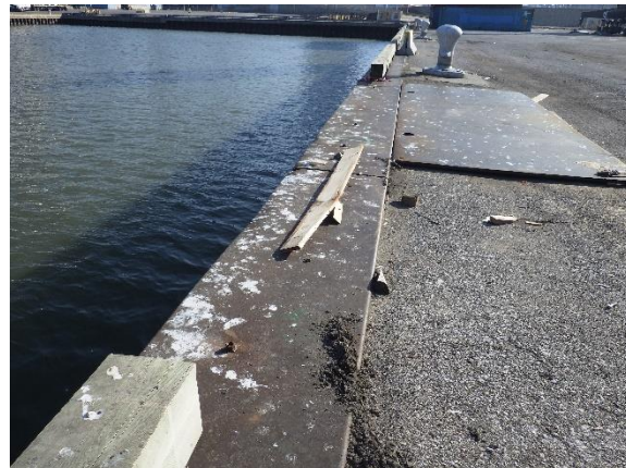
Fig. 2 – Break in timber curbing
