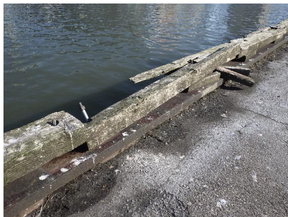
Fig. 15 – Damaged timber curbing and settled pavement
