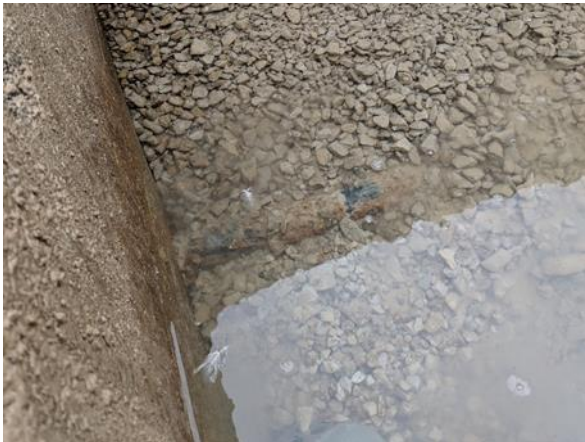
Fig. 17 – Tieback and Deadman Exposure
