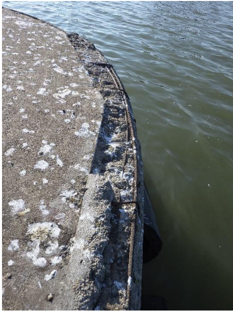
Fig. 7 – Deteriorated pile cap
