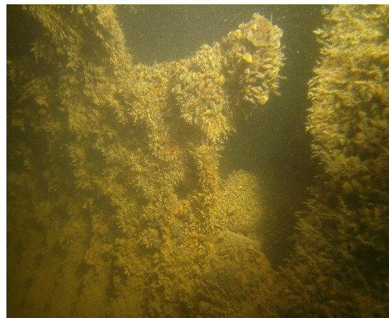
Fig. 6 – Section loss at outfall (underwater)
