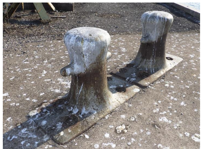
Fig. 10 – Corroded anchor bolts
