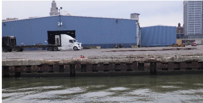
Fig. 8 – Deteriorated pile cap and break in timber curbing
