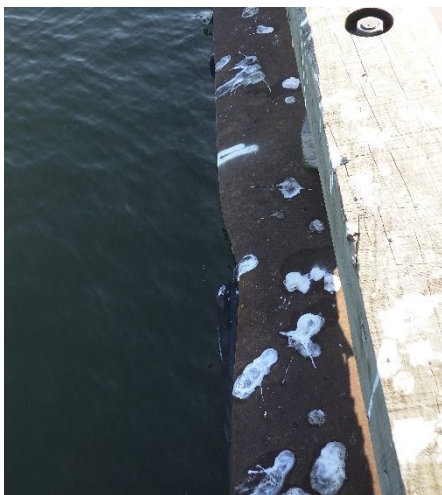
Fig. 3 – Damaged pile cap
