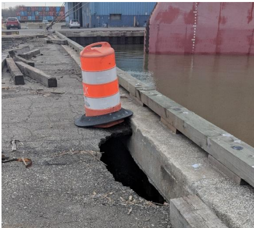
Fig. 5 – Sinkhole at CMP Outfall
