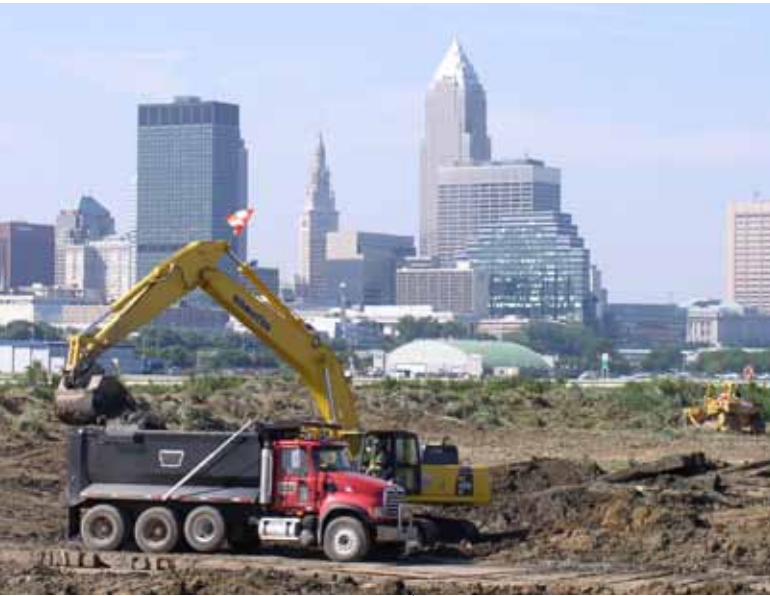
Dredged sediment from Dike 10B near Burke Lakefront Airport being removed and transported to remediate a Cleveland Brownfield site.
